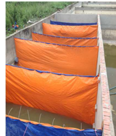
Sedimentation unit (126 m 3 )
